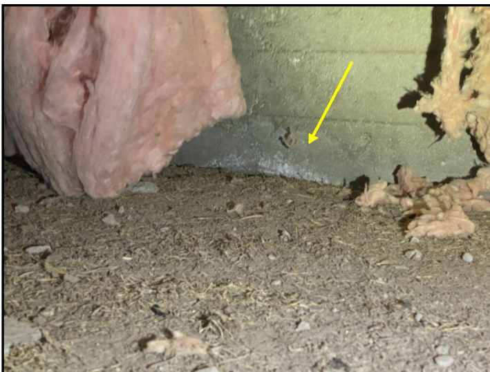
Efflorescence observed.
