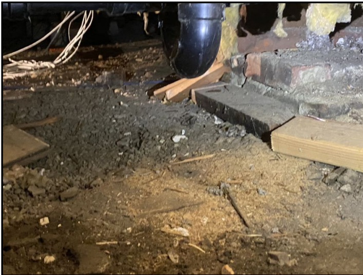
There are cellulose products in the crawlspace.
