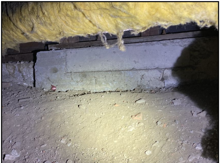
The poured concrete foundation walls appear to be functional.
