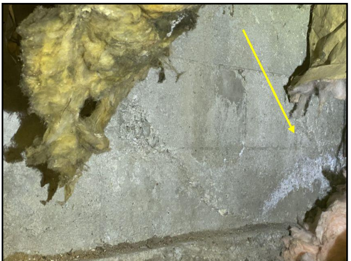
Efflorescence observed.
