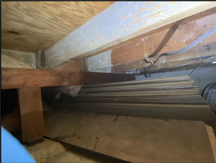
Visible areas appear satisfactory at the time of inspection.
