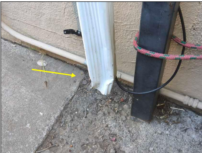
Some downspouts are missing or need to be reconnected or serviced.
