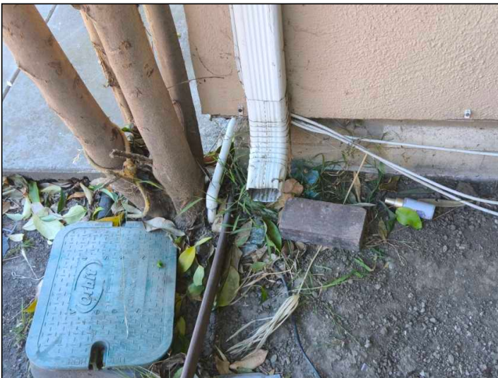
We recommend you have diverters or splash blocks installed at the bottom of all downspouts.
