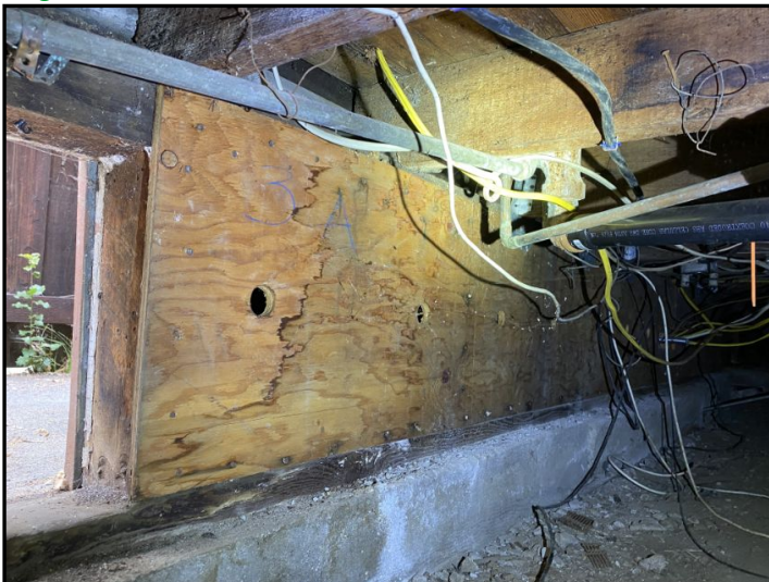
Some areas of the foundation has been retrofit with visible Plywood/OSB sheathing.
