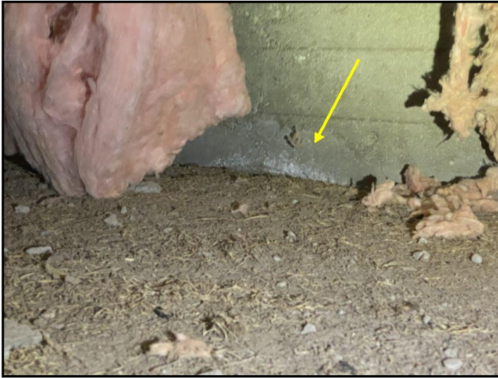
Efflorescence observed.
