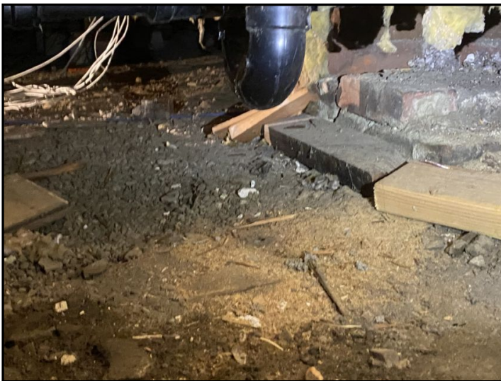
There are cellulose products in the crawlspace.
