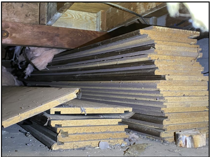
There are cellulose products in the crawlspace.
