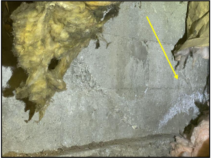
Efflorescence observed.
