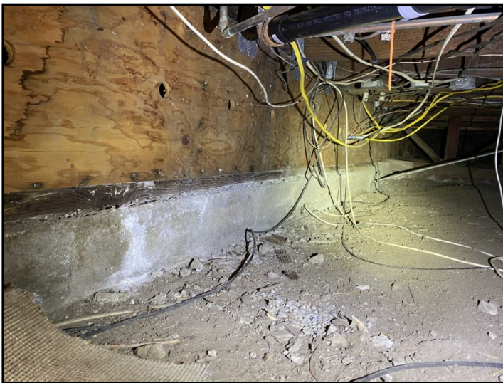
The poured concrete foundation walls appear to be functional.
