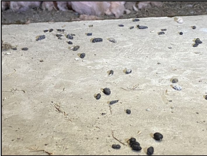
Evidence of rodent activity was observed in the crawlspace.
