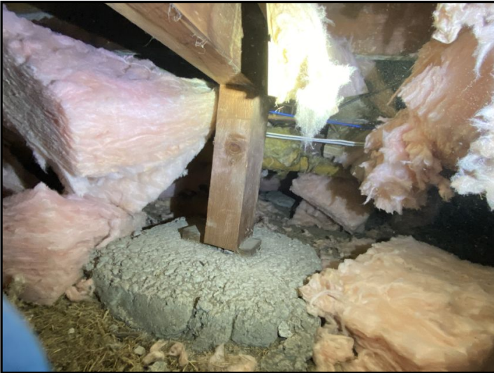
The majority of the supplemental support posts in the newer section of the property are properly placed.
