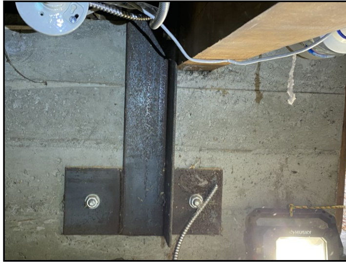
Anchor straps noted.
